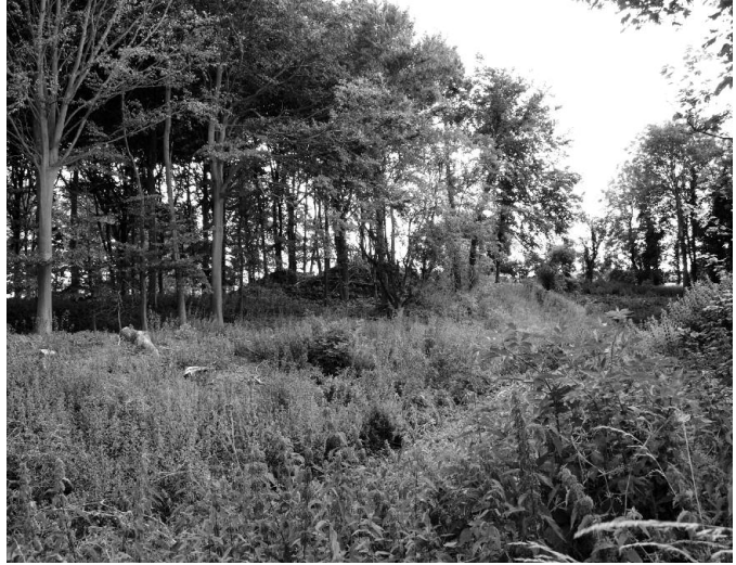
FIG. 232 – Lidgate Castle, view NE into the site from the churchyard, showing the mysterious double-peaked feature on the SE corner of the castle platform.
